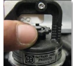
Figure 2 Pressure Switch Adjuster
